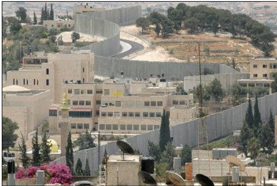
Figure 8: The Barrier is an additional impediment to Palestinian movement. A 703km long complex series of 8-9m high concrete walls, electronic fences, observation towers, trenches, patrol roads and razor wire used to block Palestinian pedestrian and vehicular movement inside the West Bank and East Jerusalem.
