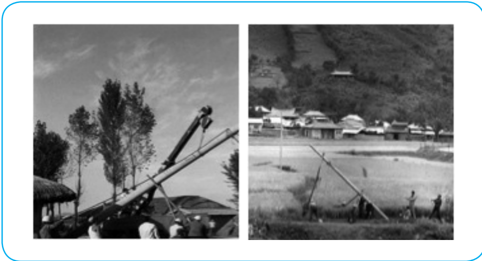
Figure 1-1 | Rural Electrification Project
