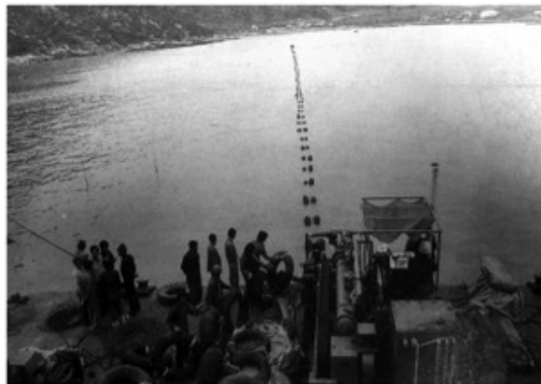
Figure 2-5 | Electrification Project Construction (Installation of Submarine Cable)
