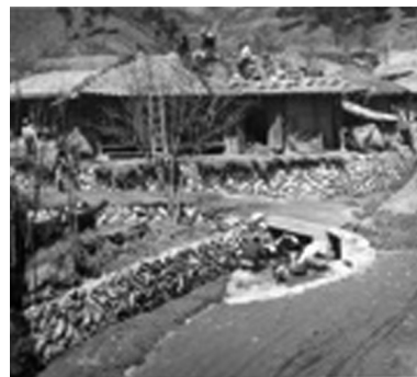
Renovation of rural house roof in the 1970s
