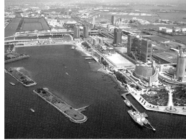
Seaside Sub-center, Tokyo, Japan
