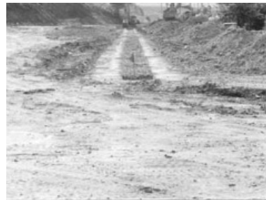
Bentonite Upper Covering for Impermeable Wall
