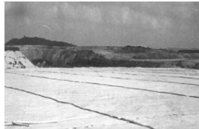
Spreading Non-woven Cloth
