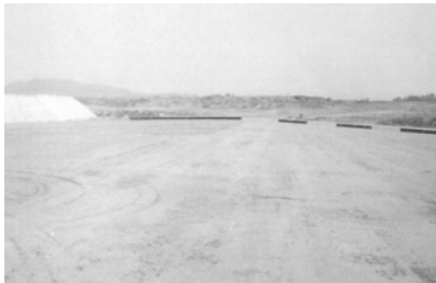
Paving the Support Layer
