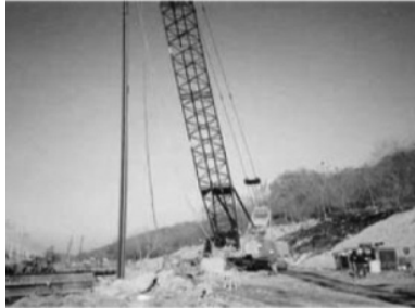
Sheet Pile Transport for Impermeable Wall Support
