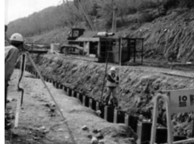
Installation of Sheet Pile for Impermeable Wall Support
