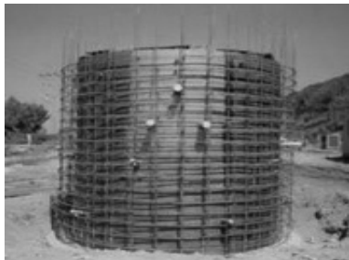
Production of Leachate Collection Wall
