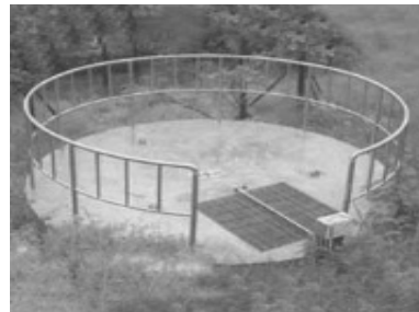
Completion of Leachate Collection Well
