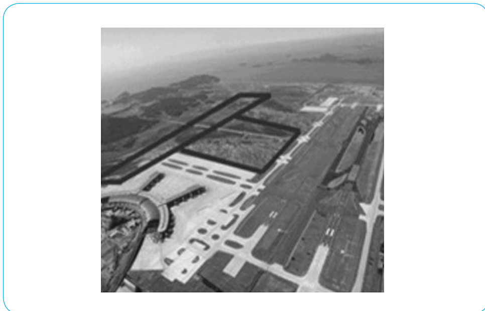
Figure 5-6 | Construction Site of Incheon International Airport at Phase 2
