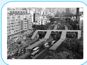
Figure 5-2 | View of BRT Station
