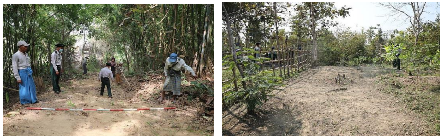
Figure 14. Preparation of fires road on community forestry (Quarterly Report, 2022)
